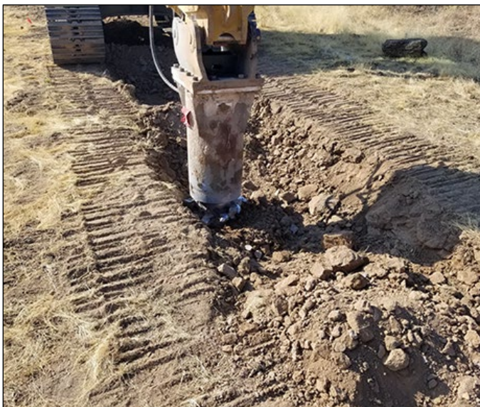
A vertical grinder was used to grind out the fence posts.
