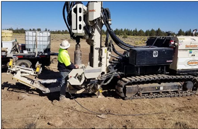
Below-ground fence post removal using a track-mounted Geoprobe sonic drill rig.
