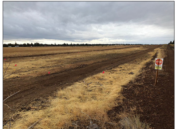
A section of Tulelake AFS after fence post removal and backfilling.
