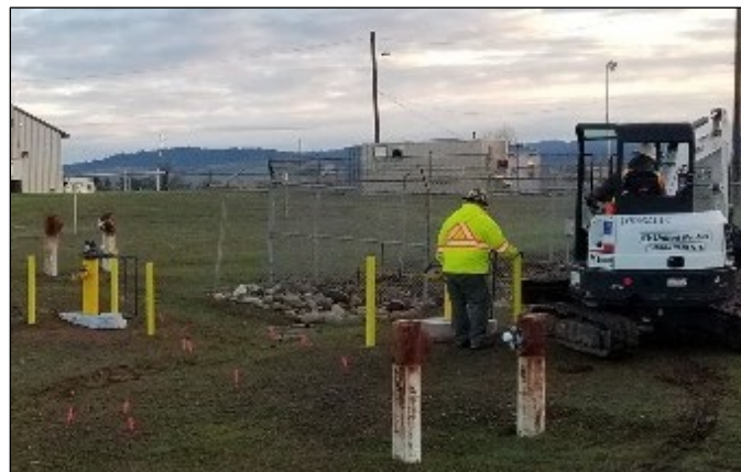
Pipe installation at a sparge well with the biosparge system in the background.
